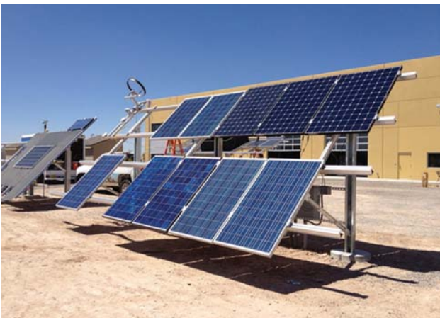
Solar modules undergo testing at OTF-1 in Albuquerque, NM
